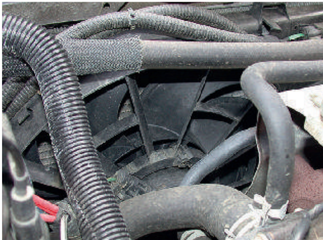
Figure 3.163 Condenser cooling fan
